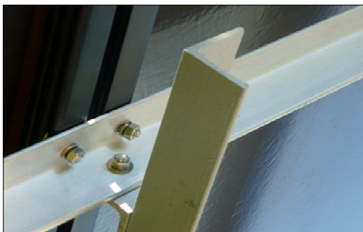
Figure 2. Attach Panel Kit Rail to Cross Rail using L-Bracket.
