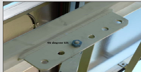
Figure 3. How to Adjust PV Array Tilt Angle.
